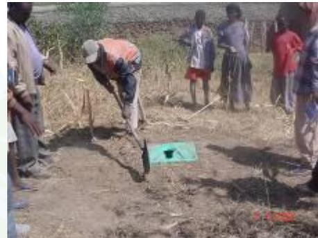
The slab is placed on the pit after excavation
